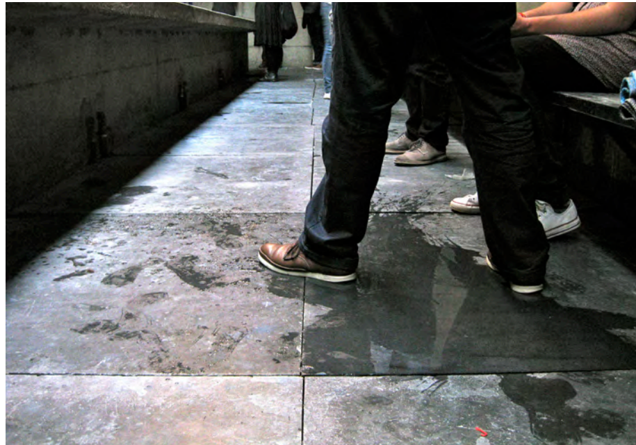
Water on the floor transforming the slate from a matt to gloss surface.
