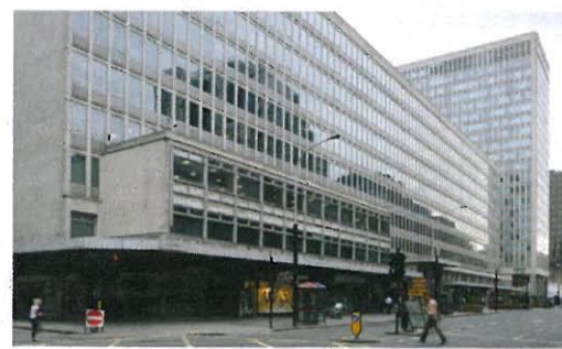
The existing Kingsgate House on Victoria Street dates from the 1950s.
